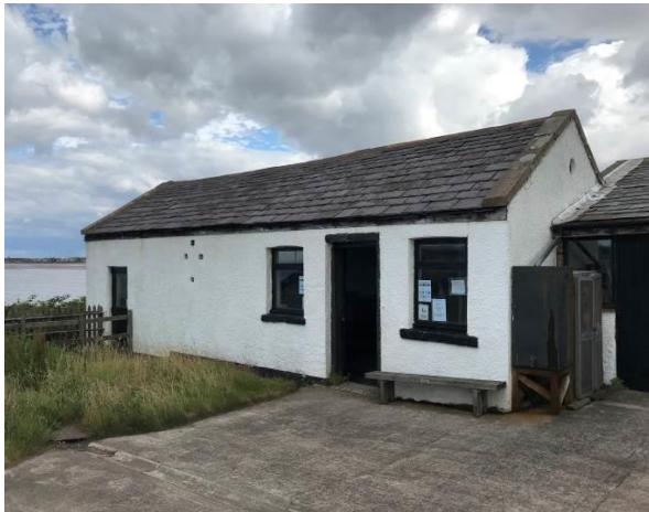
Day/School Room north elevation
