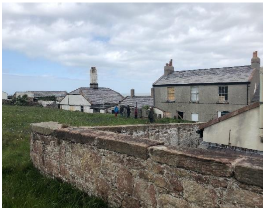
View of the Buoymaster's House
