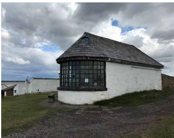
Telegraph Station viewed from north-west
