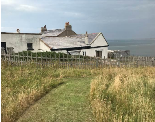
Bouymasters Store, south elevation, two storey part to left
