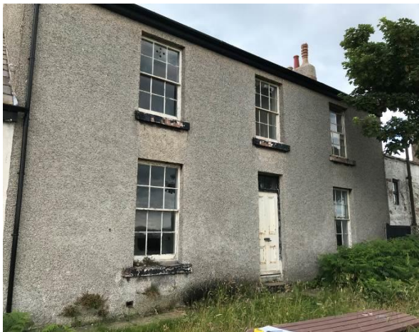
Bouymasters House front (east) elevation
